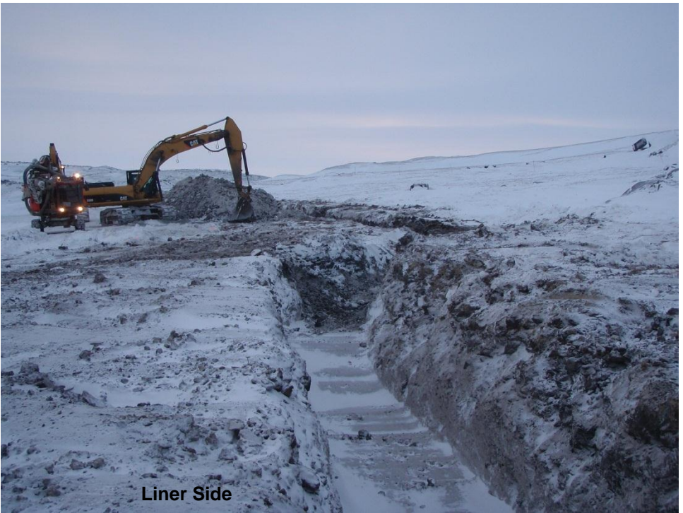
Photo 10: Doris North Diversion Berm. In some areas, the key-trench requires significant cutting to achieve a slope acceptable for liner placement. Photo looking west towards Quarry 2.
