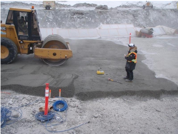
Photo 4: FCM placement over top thermistor cable DN-HTS-130-31.0; only static compaction was used directly above the cable.
