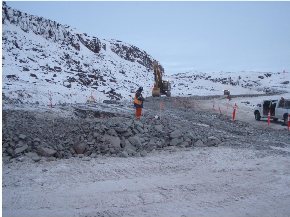
Photo 7: ROQ placement at the Doris North Diversion Berm. Note the packer (in the background) has been mobilized to compact ROQ between lifts.
