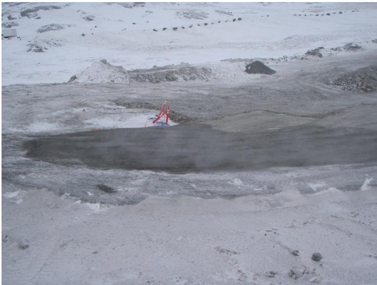
Photo 6: Small additional patch of FCM placement at the southwest end of the dam.
