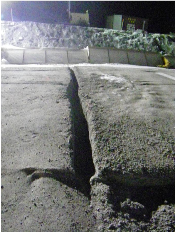
Photo 14: Trench cut in FCM at 1+75 to allow for installation of the next horizontal thermistor at the correct elevation.
